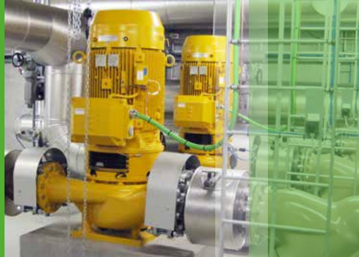
Space saving installation with vertical NSL pumps.
