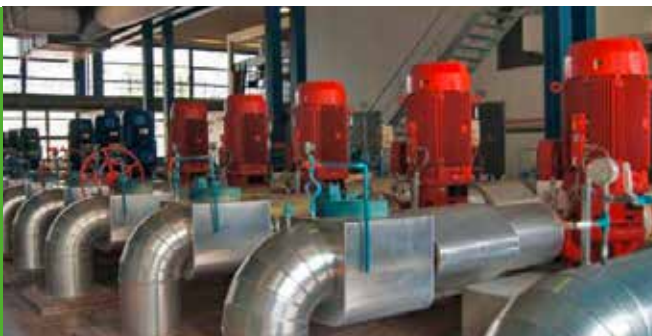
Vestforbrænding, Waste-to-Energy Plant, Copenhagen DESMI supplied many pumps to this facility: 12 x NSL 200-415B/A12 + 200 kW, 2 x NSL 200-415B + 200 kW, 2 x NSL 200-415B + 200 kW & 5 x NSL 125-330 + 110 kW
